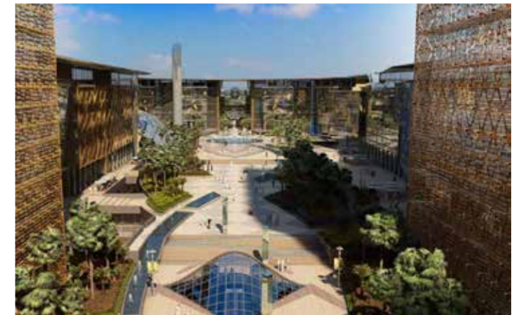
ITCC CONVENTIONAL TOWER (Riyadh, Saudi Arabia)
