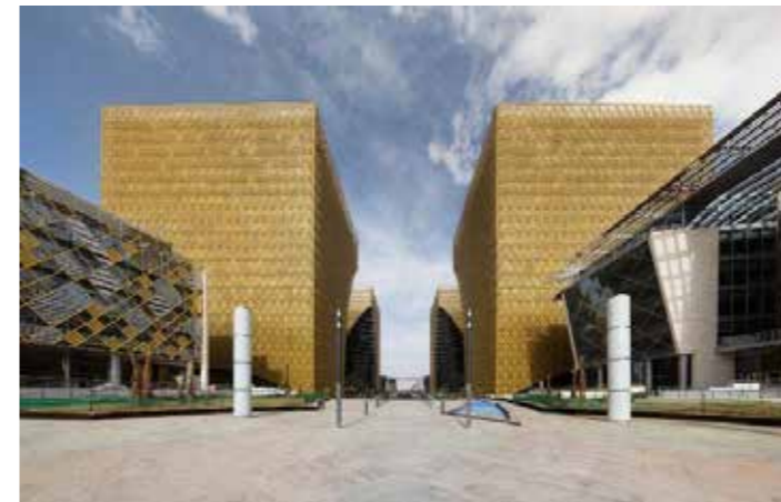
ITCC CONVENTIONAL TOWER (Riyadh, Saudi Arabia)
