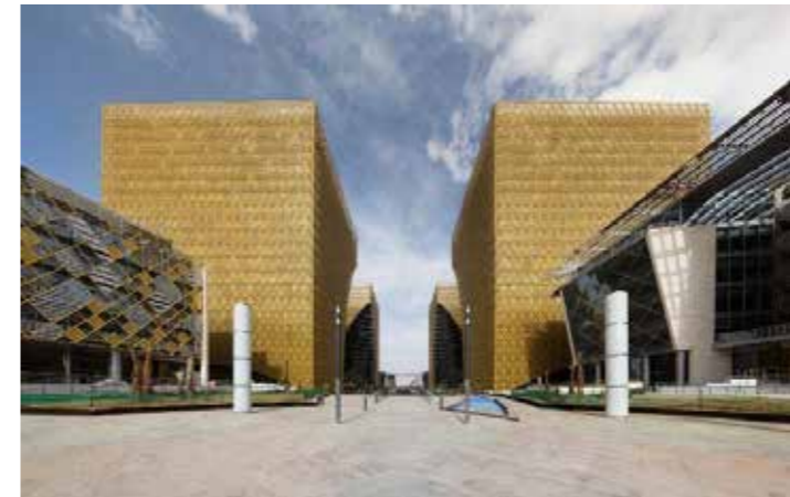
ITCC CONVENTIONAL TOWER (Riyadh, Saudi Arabia)
