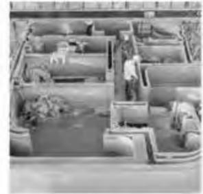
The **BOD2** printer is the fastest and highest quality 3D construction printing system in the world. Using this technology along with additive materials developed by **COBOD** and their partners at **CEMEX**, the **BOD2** is capable of printing using local concrete materials. This ensures a significant reduction in cost as well as construction time.
